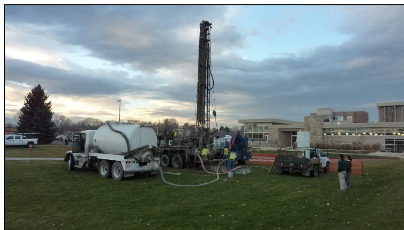
Drilling a test well to determine conductivity in the soil
